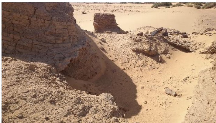
Fig 6. Roman house located to the south of Tulieb fort, has been attacked by the robbers in 2013. Photo by the author (2024)
