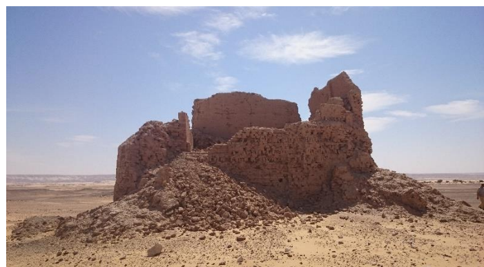
Fig 4. The piles of mudbricks that brought out of the fort by the robbers. Photo by the author (2024)
